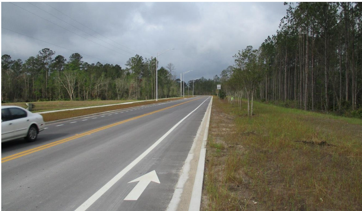
Newly constructed road: New World Avenue (facing west)
